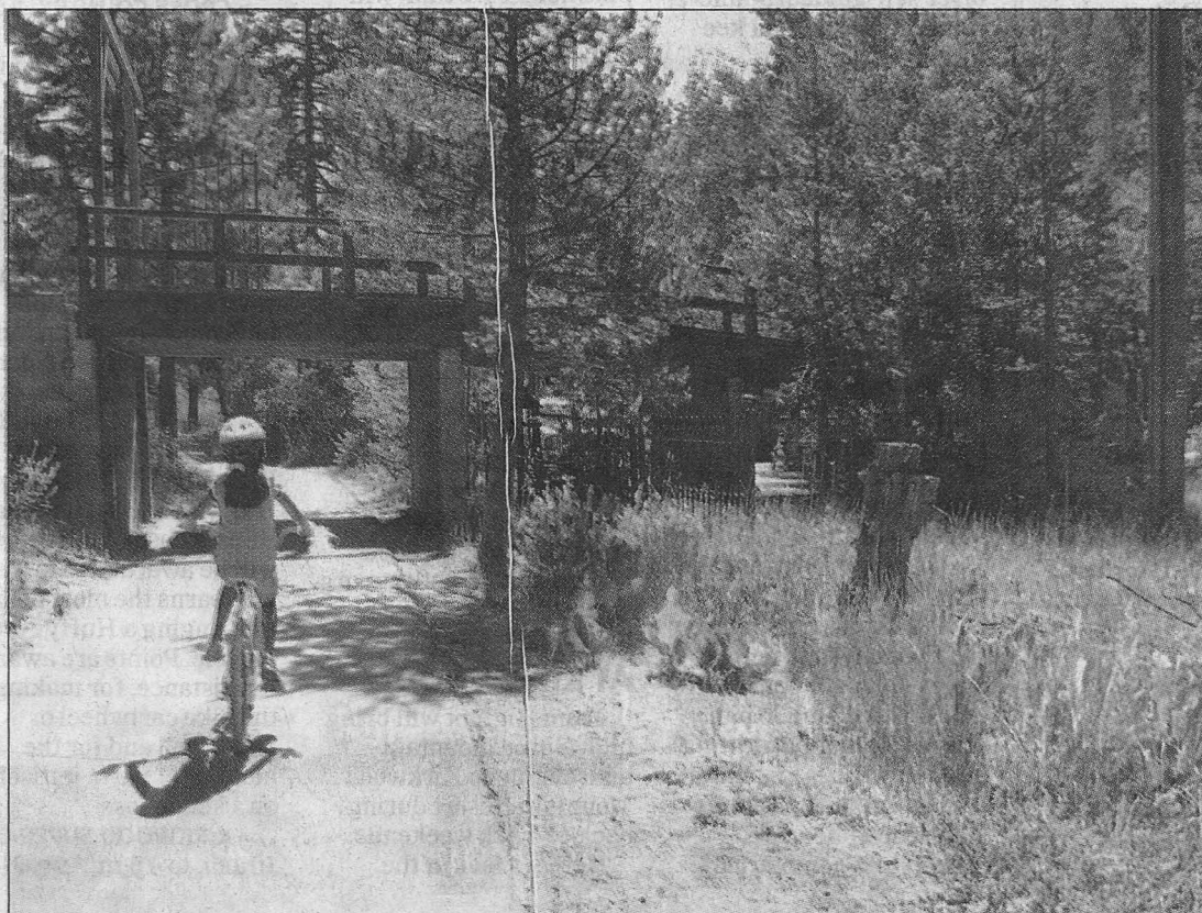
An old wooden bridge is part of the scenery along the Tahoe-Pyramid Bikeway between Squaw Valley USA and Tahoe City. The well-maintained trail is about five miles one way. JACKIE GREEN/RGJ
